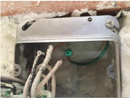
This picture was taken of an electrical box at the Arbor Trails Senior Housing on Blairs Ferry. It shows insulation sprayed into the outlet box, which is a violation of the Electrical code not allowing foreign (non-approved) materials in any electrical installation. The insulation company should have covered them before spraying. Since they didn't they had to go back and clean the combustible material out of each box.
