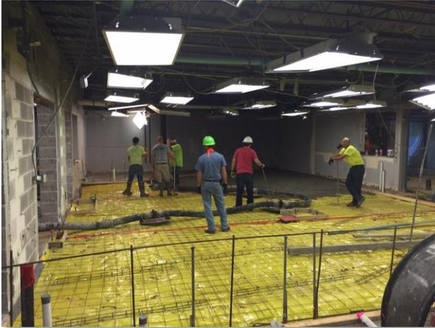
Contractor pumped concrete over 300' to pour the Linn Mar Kitchen floor. You can see the hose laying on the floor.
